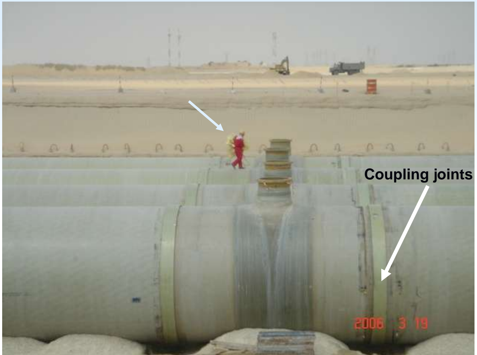
500 mm (20" ) air valve connection on 4M pipe
