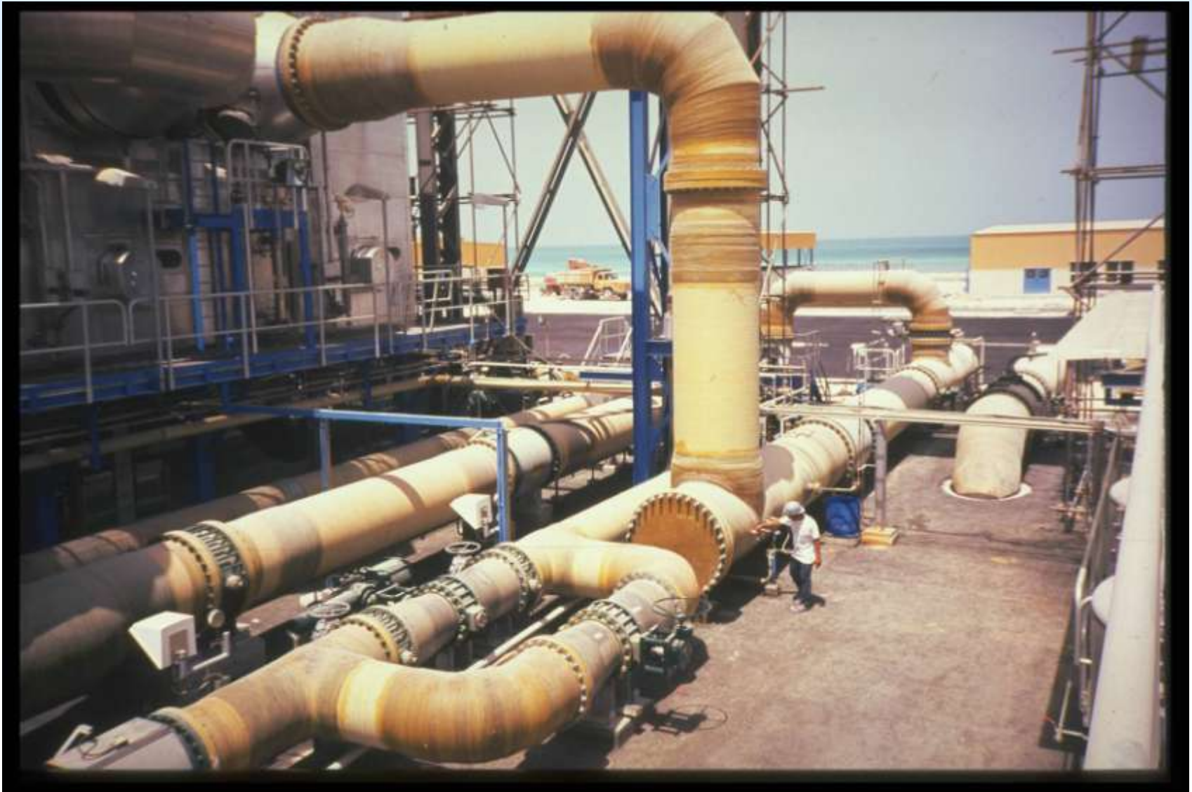
Jebel Ali G station – 1200 mm GRP Product water at MSF evaporators
