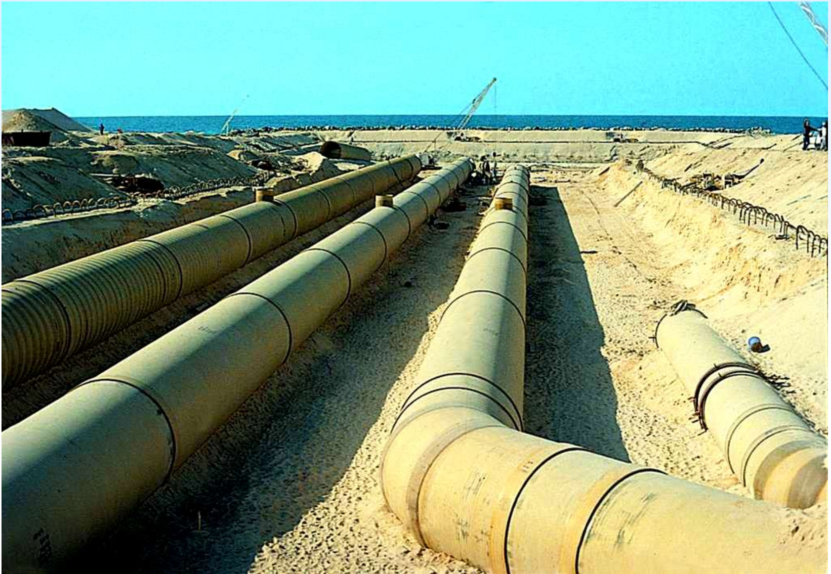
2.4m supply & 2.7m Return Pipe – Jebel Ali G station 270,000 M3/day-1992
