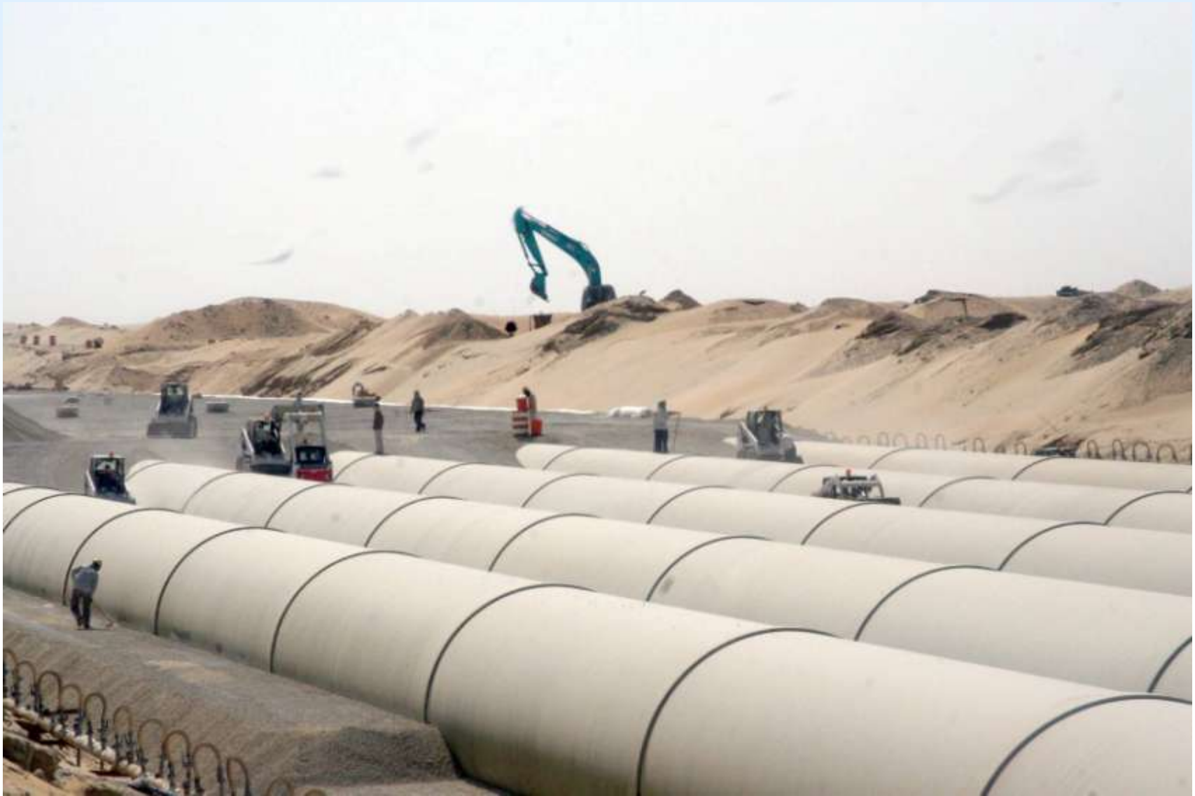
Bobcats being used to place backfill on sides on pipe
