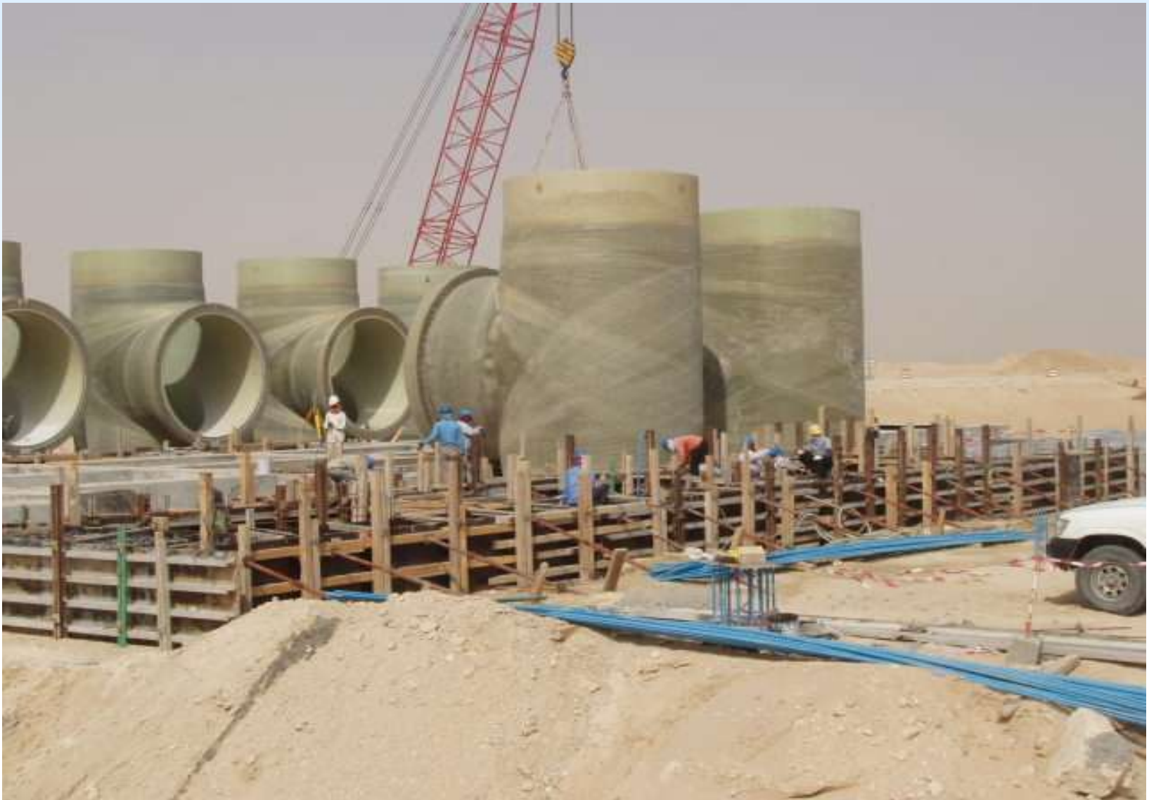
4M Equal Tee with Flanged 4M Branch on site
