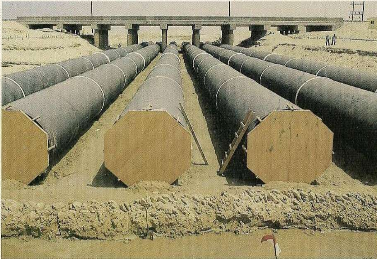
This section of the Jubail Industrial City seawater cooling system in Saudi Arabia utilizes six barrels of 1600-mm-diameter prestressed concrete cylinder
