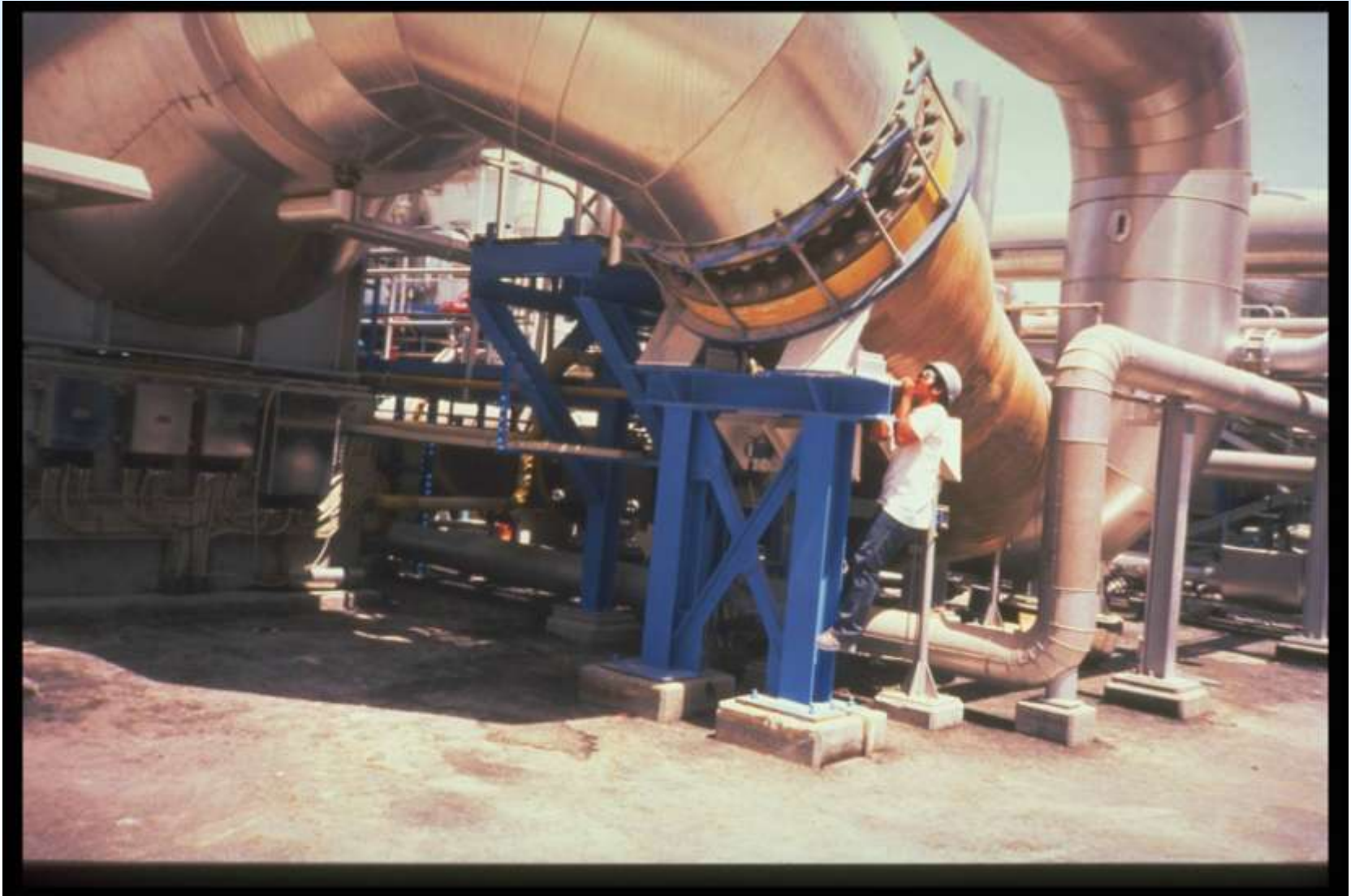
Jebel Ali G station – 1800mm GRP Sea water supply piping to MSF evaporators
