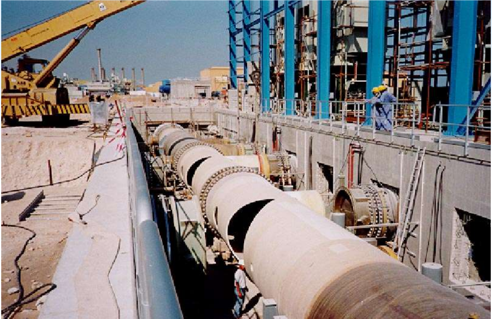
Main Sea Water Pump House Header 2.5 mm dia. Length = 66M
