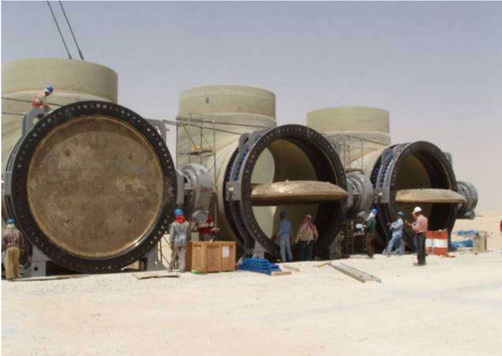
4M Butterfly Valve Installation
