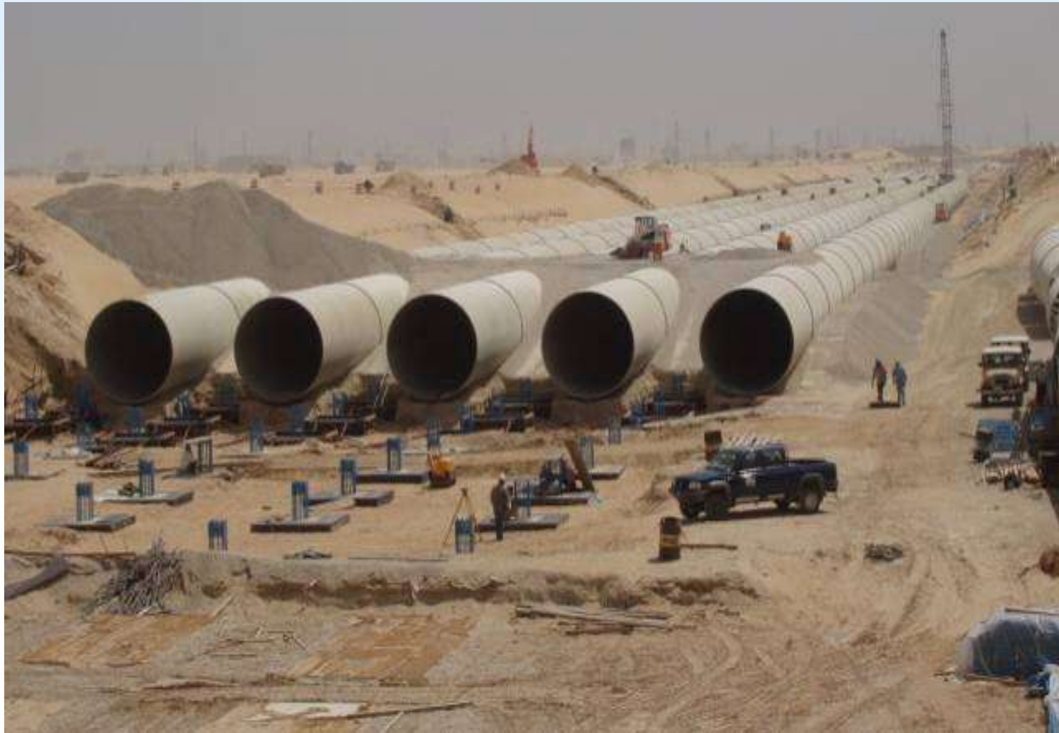
5 Barrels of 4.0M pipe installed in 34M wide common trench
