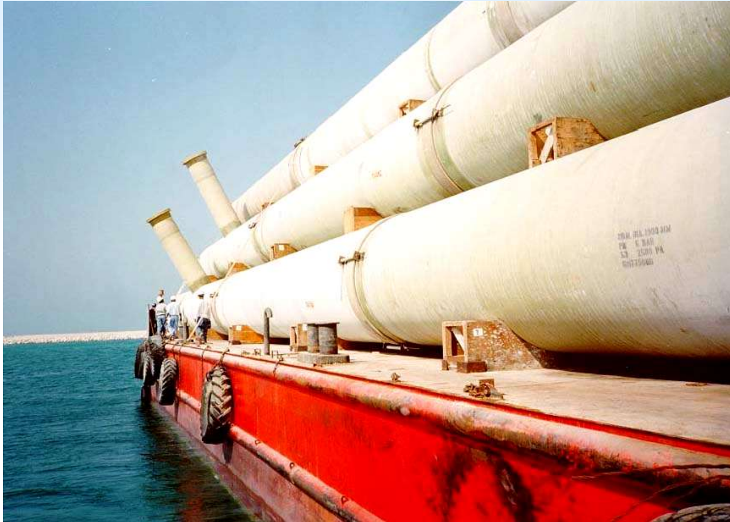
1.9M Intake Pipe L=36M – Ras Abu Fontas B (ABB) On barge – Notice DN 900 mm flanged access man-ways
