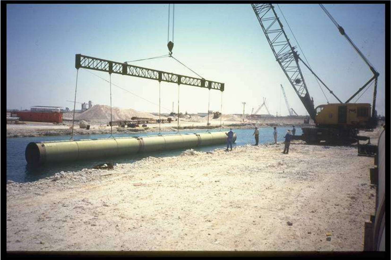
Ras Abu Fontas B (ABB) Offshore Installation– 36M Pipe sections pre-assembled onshore
