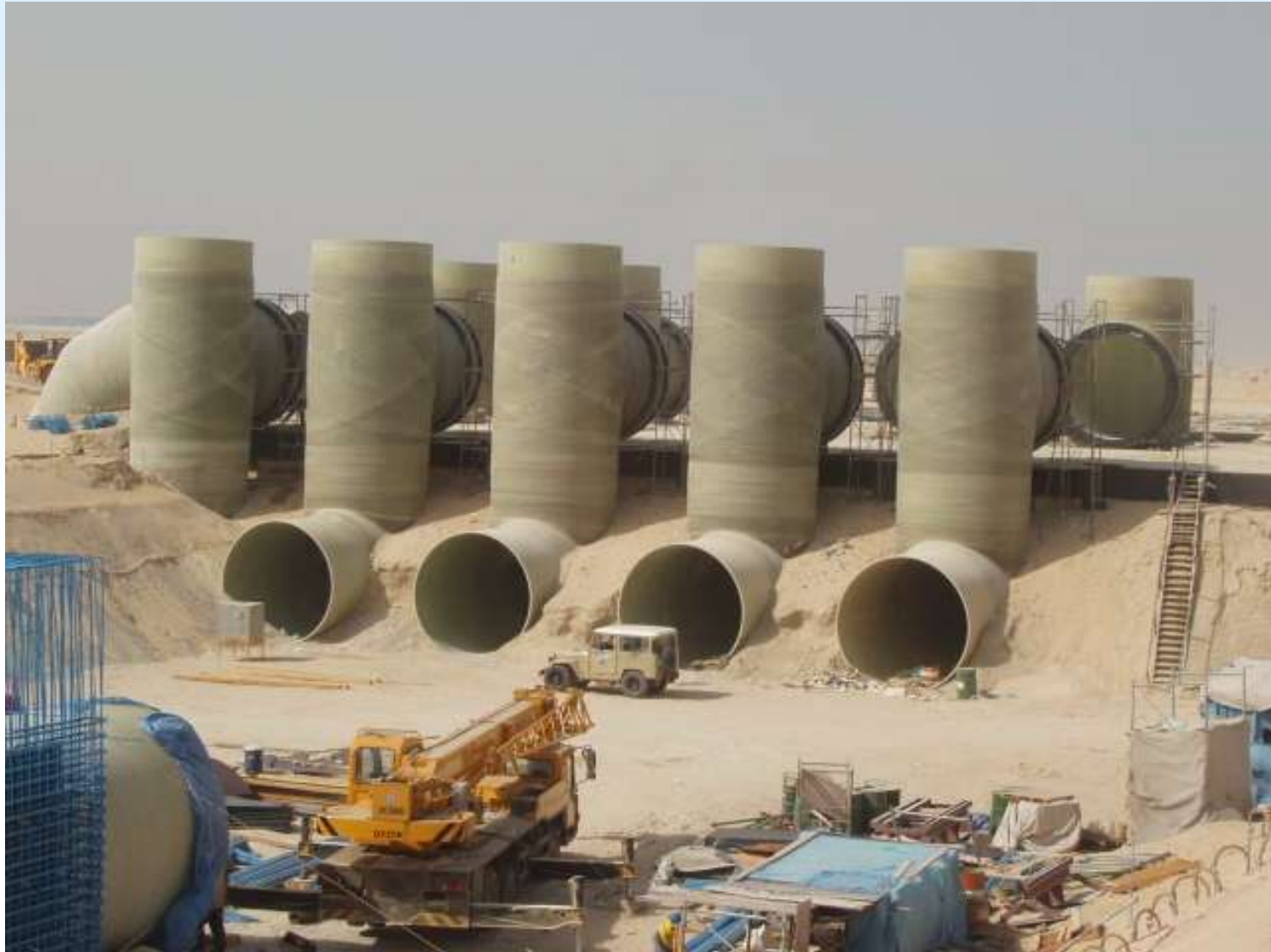
4M Equal Tee with Flanged 4M Branch on site
